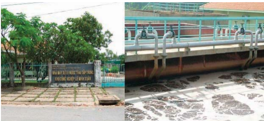
The picture presents the sewage treatment station in Le Minh Xuan industrial park
