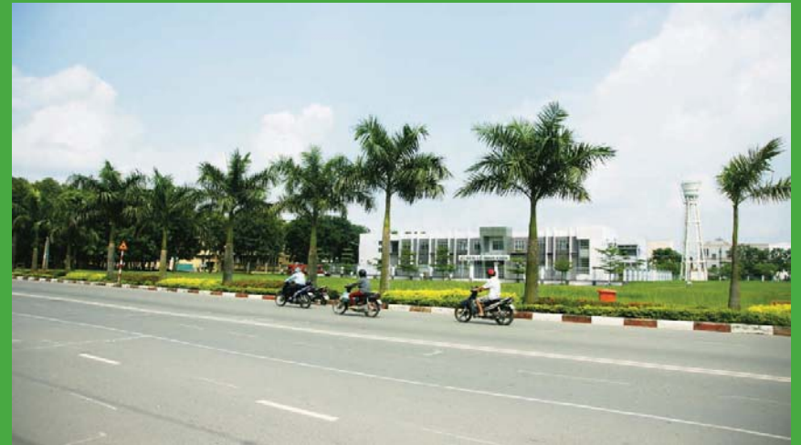
Le Minh Xuan industrial park's access route
