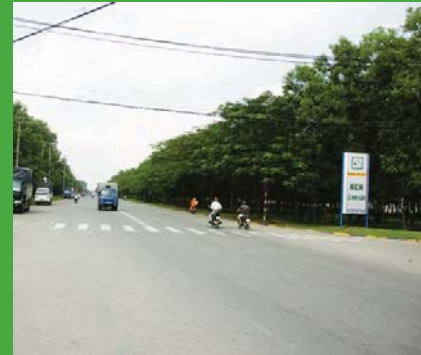
Le Minh Xuan industrial park's access route
