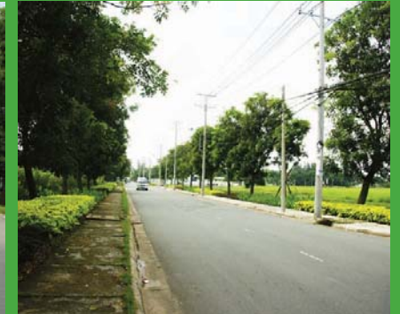
Le Minh Xuan industrial park's internal route
